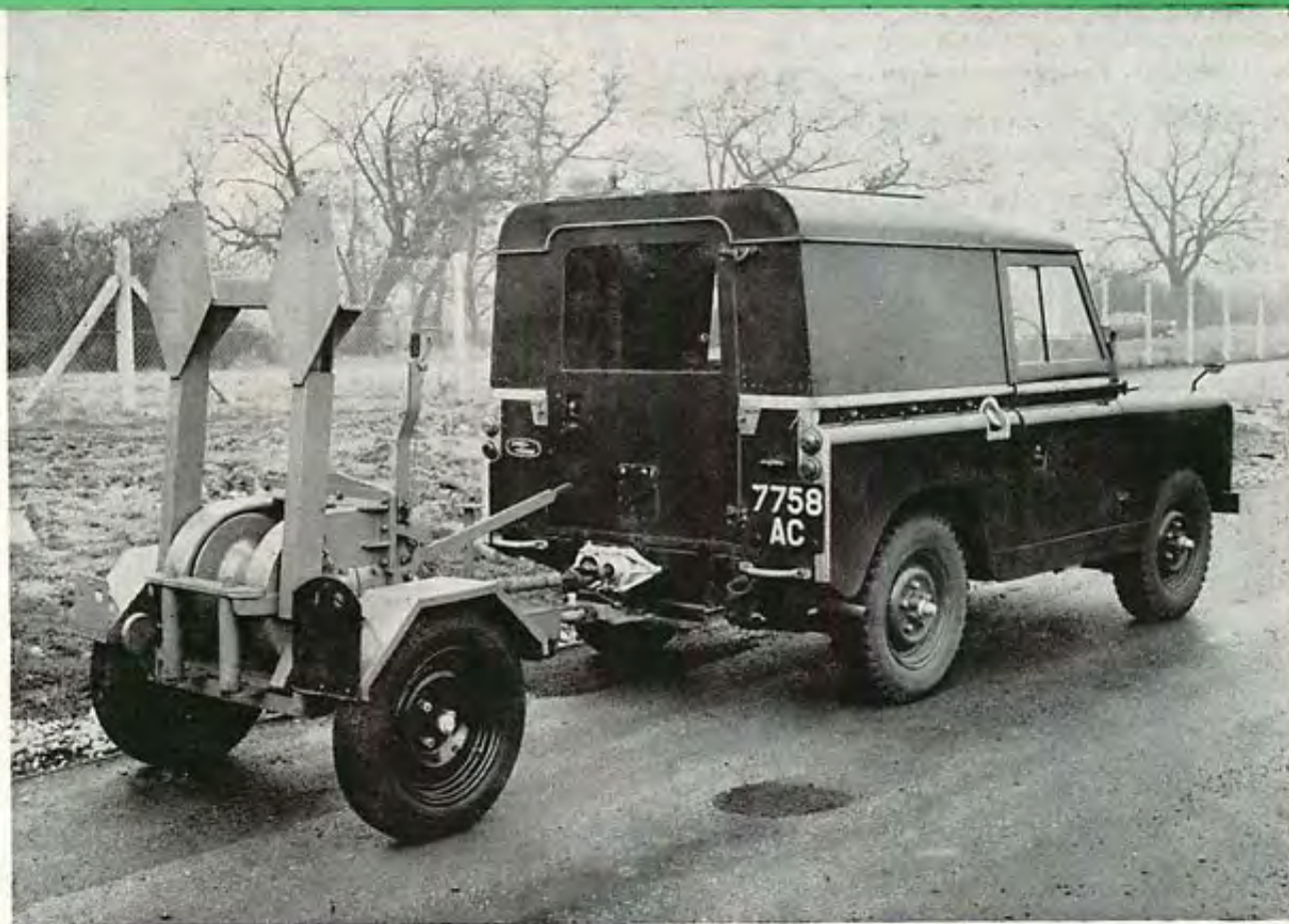
The Hesford Trailer Winch attached to the Land Rover with the anchor in the transportation position.
