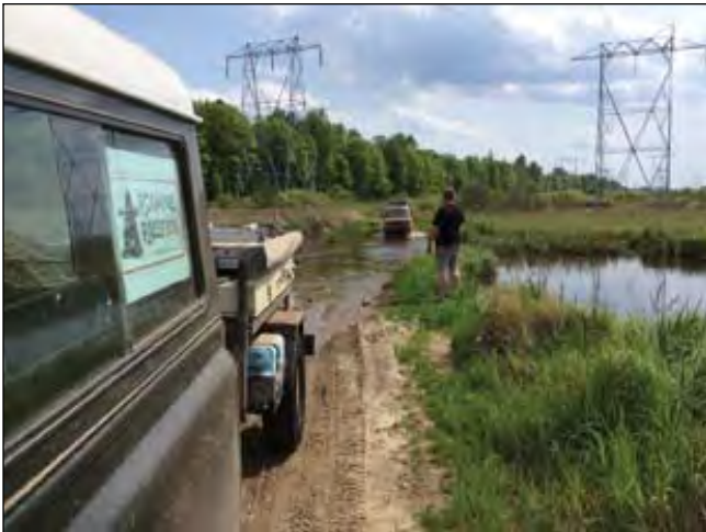
On a hydro line near Calabogie.
