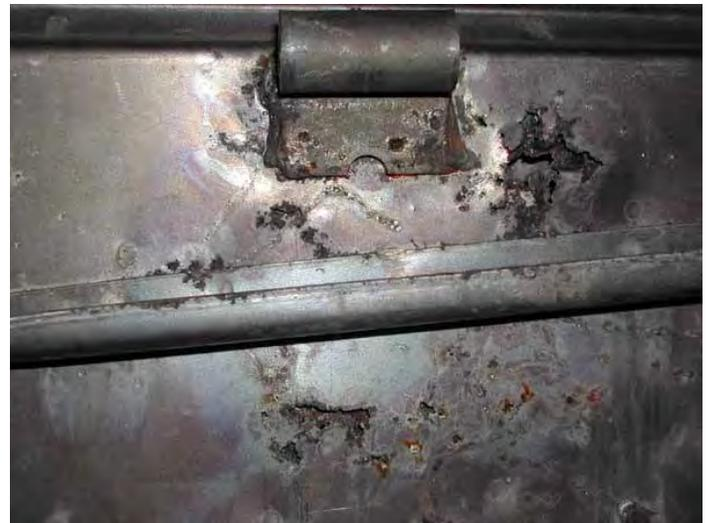
(Figure 1) This is typical upper bulkhead rot. Hearsay will tell you this is a difficult repair when in reality its quite simple to make a quality repair here. The key is the removal of the hood hinge and drip rail and support bracket. Then an effective repair can be made with a conventional replacement panel. Measure and record the placement of the hinge and support bracket on the firewall and then carefully grind away the welds securing them to the firewall. Then drill the spot welds
