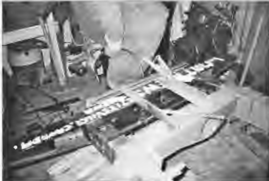
New rear cross-member held in place by jig ready to be welded.
